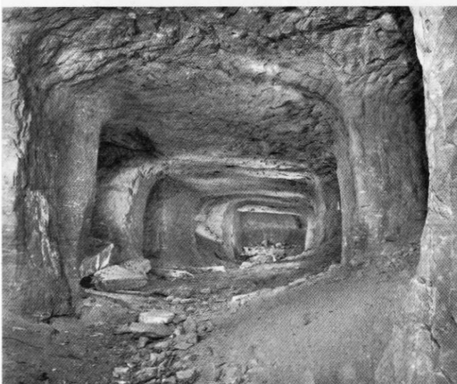
Looking east along one of the galleries. Note the rock bed dips down to the south. The nearly flat ceiling profile reflects the flat lying iron-cemented bed immediately above the mined sand. Floor to ceiling height at this point is approximately 2 metres. Photo by Nick Catford
